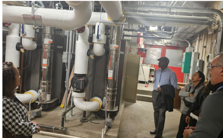
Board of Education members toured District buildings to see the status of Capital Projects.
