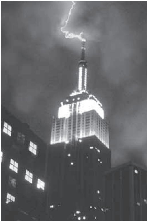
Lightning strikes the lightning rod rather than the building, because the lightning rod is the tallest point on the building.
