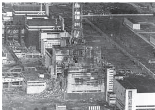
During a test at the Chernobyl nuclear power plant, the emergency protection system was turned off. The reactor overheated, causing an explosion.
