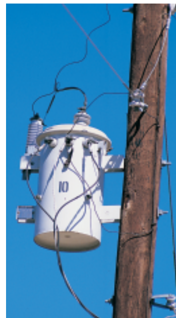
FIGURE 25–13 Step-down transformers are used to reduce the high voltage in transmission lines to levels appropriate for consumers at the points of use.
